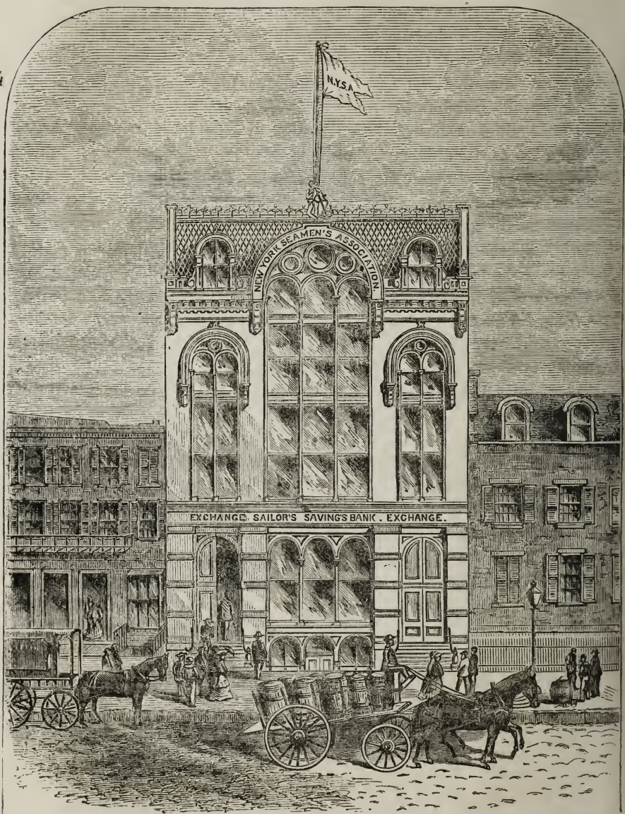
NEW YORK SEAMEN'S EXCHANGE BUILDING.
